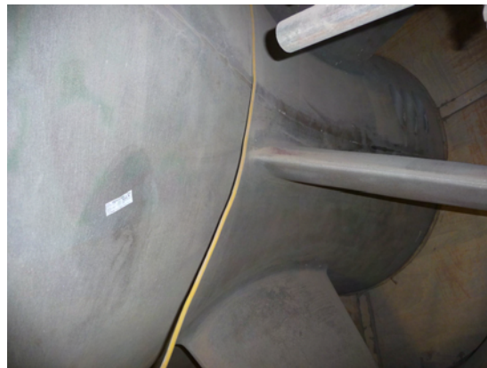
Picture 2 – Bellmouth after grit blasting
