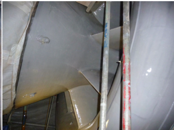
Picture 4 – completed coating RS 500P
