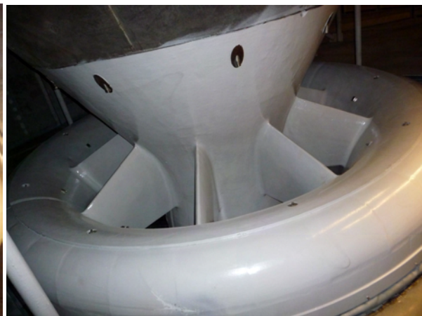
Picture 6 – Completed topcoat RA 500M
