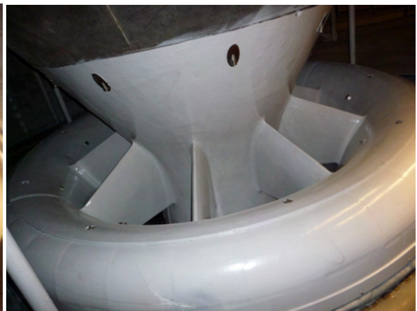
Picture 6 – Completed topcoat RA 500M
