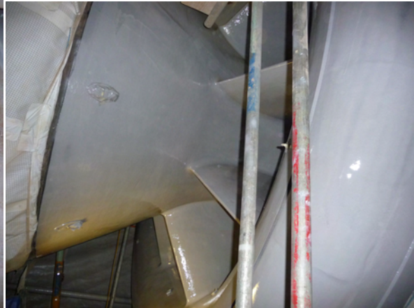
Picture 4 – completed coating RS 500P
