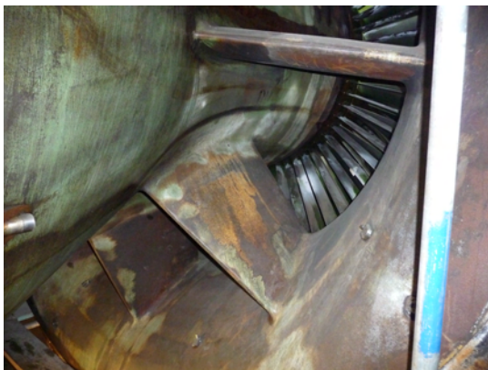
Picture 1 – Bellmouth prior to coating
