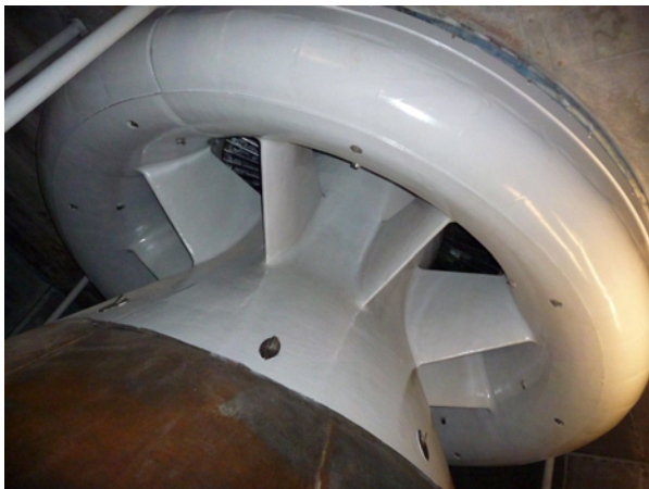
Picture 5 – completed topcoat RA 500M
