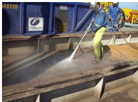
Wet abrasive blasting
