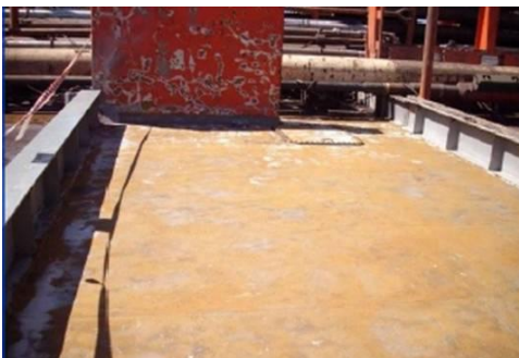
Corroded deck
