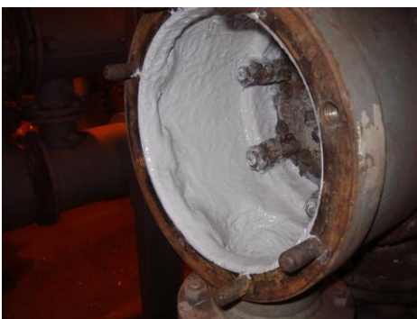
Water boxes after W/B, priming and application of RA 532
