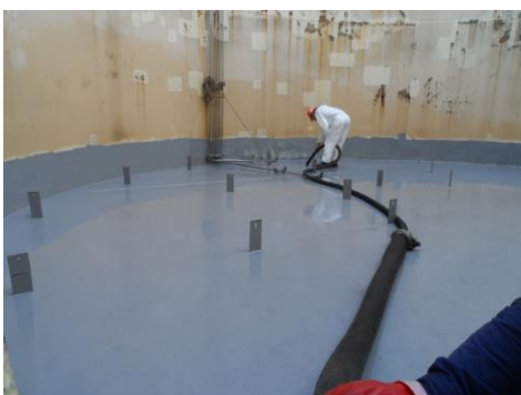
Preparation of top coat
