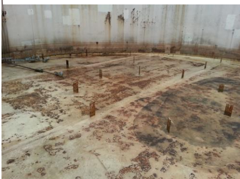
Corroded Floor
