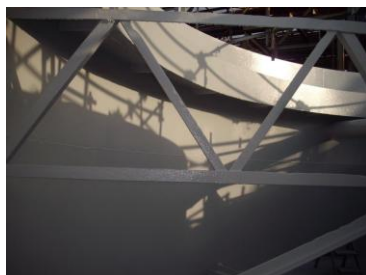
Launder and steelwork
