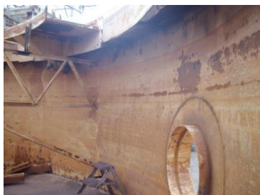
Before – Clarifier on inspection
