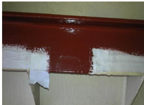
Application of RS 500P a wet & rust tolerant primer
