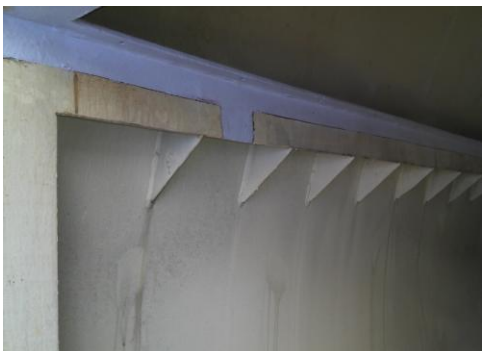
Application of RA 532 a wet tolerant glassflake filled epoxy
