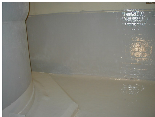
Epo-chem™ RF 500 Bund Lining
