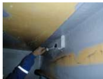
Applying RA 500M on wet surface
