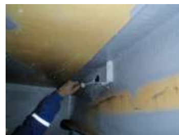
Applying RA 500M on wet surface
