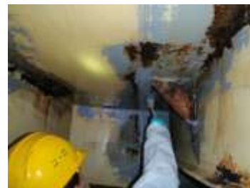
Applying RS 500P on wet & rusty surface
