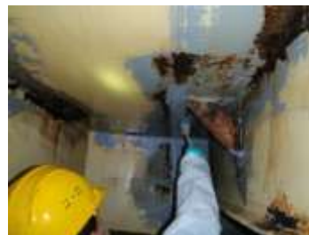
Applying RS 500P on wet & rusty surface
