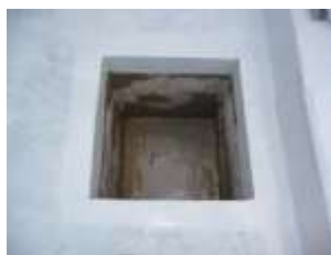
Chem-concrete™ RJ 800CRS Chemical Sump Repair
