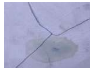
Chem-concrete™ RN 800CRS Crack Repair
