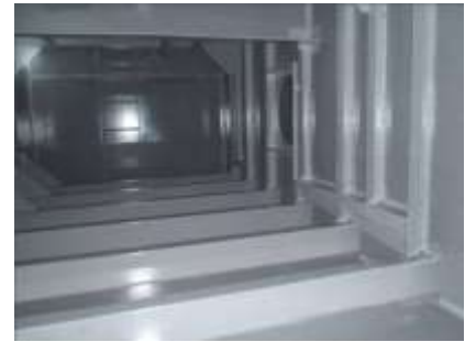
Potable Water Tank
