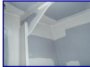
All sharp edges, corners and weld areas are coated with RA 500M
