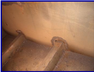
Acceptable mechanical preparation standard
