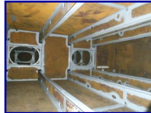
All sharp edges and corners are coated to a minimum of 100µ
