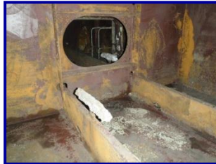
Acceptable water jetting preparation standard
