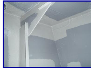
All sharp edges, corners and weld areas are coated with RA 500M
