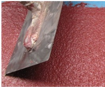
Applying InD-Cote™ by trowel
