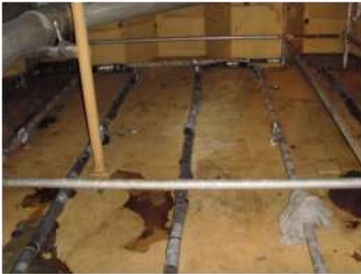
Chemical tanks before cleaning and surface preparation
