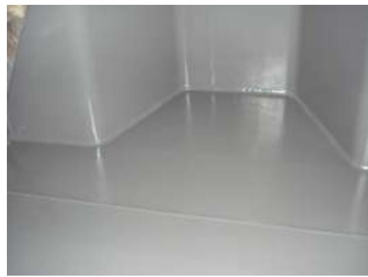
Epo-chem™ RW 500: Topcoat / Second Coat
