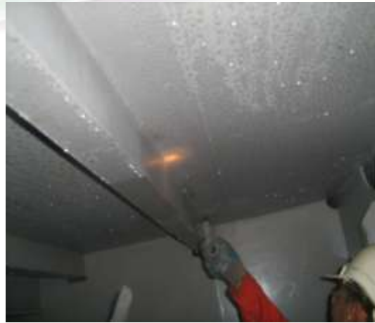
Applying Epo-chem™ RA 500M on a wet surface
