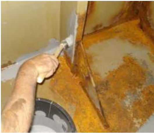
Applying Epo-chem™ RS 500P on a rusty surface
