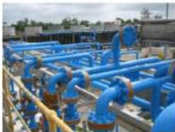
After – Coated Pipework
